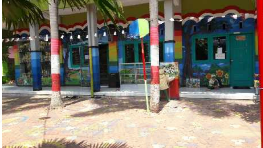
J.1 Gedung TK ABA 1 Kaliwates
