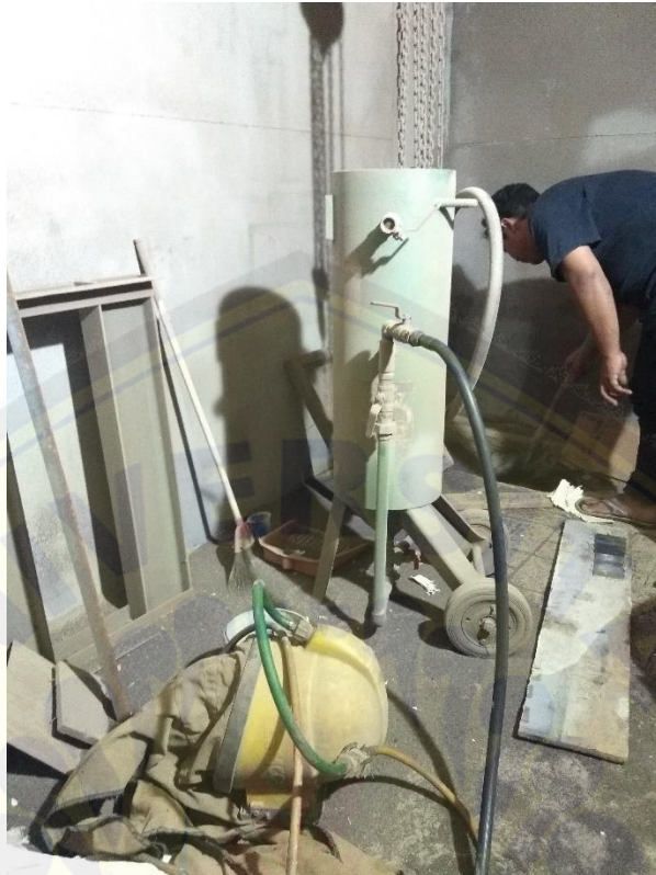
Ruang grit blasting
