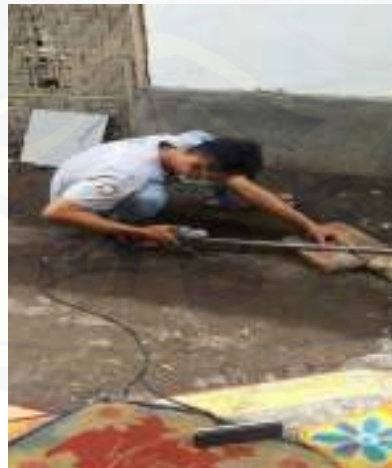
Gambar 3.4 Pemotongan pipa stainless
