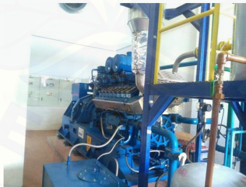
Gambar 2. 11 Generator Biogas
