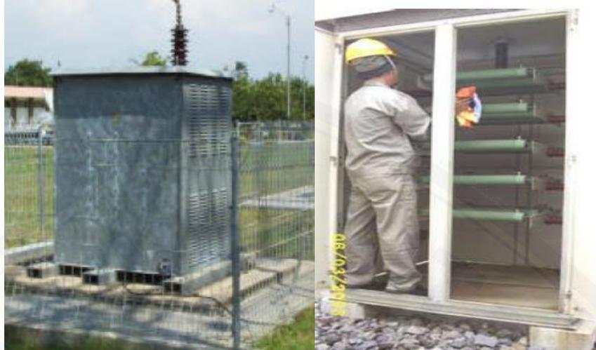
Gambar 2.8 NGR ( *Neutral Grounding Resistor* )
