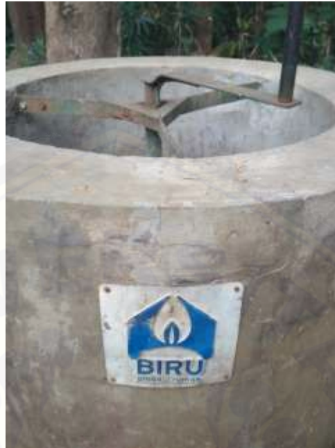
Gambar D.1 Reaktor Biogas
