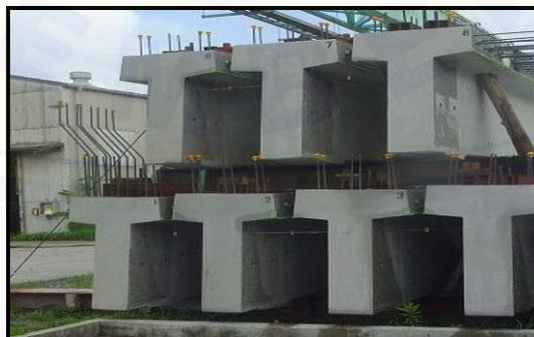
Gambar 2.5 Balok girder tipe PC-T (Sumber : www.iandengineering.com )
