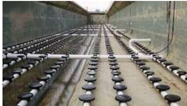
Gambar 2.5 Diffuser air systems aerator (Sumber : www.indimart.com )
