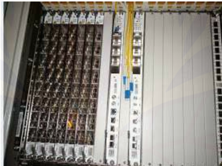
Gambar 2.7 OLT ZTE PT. Telkom Indonesia
