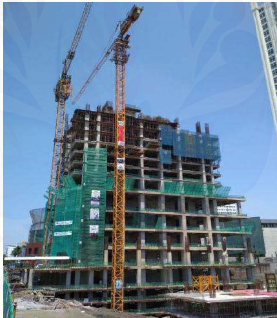
Gambar. 3.2 Tower Caspian Grand Sungkono Lagoon (Dokumentasi, 2018)
