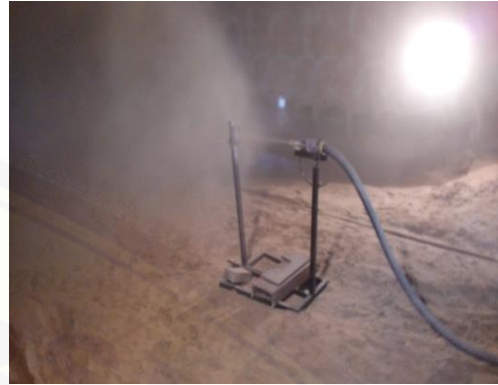
Pross sand blasting
