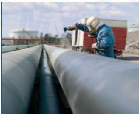
Gambar 2.1 Proses Sand blasting
