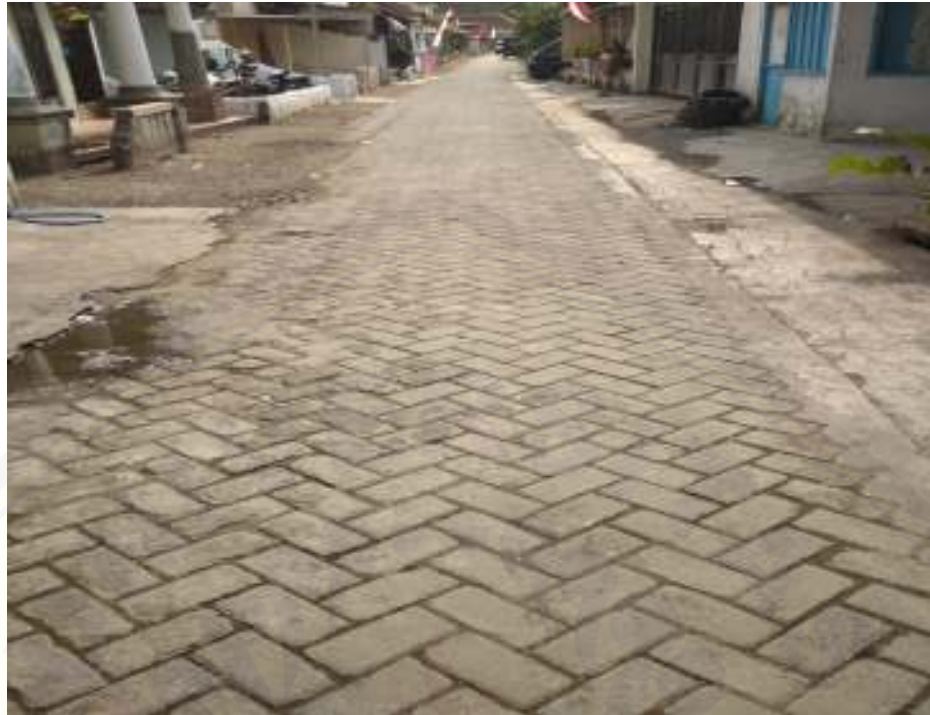
Gambar 7: Jalan Paving Rw 02
