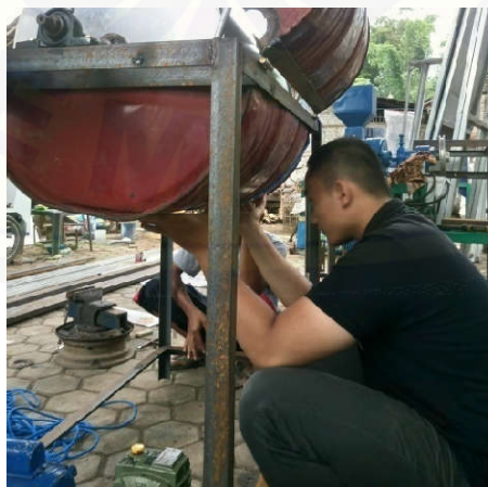
Gambar C.17 Proses Pemasangan Drum Penutup
