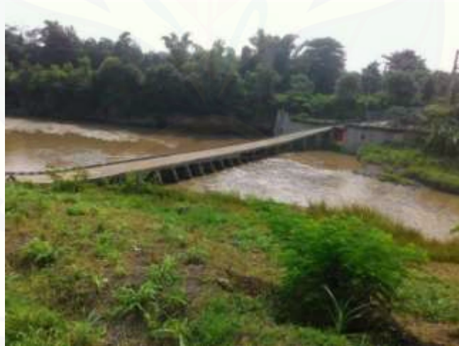
Gambar 1.1 Jembatan Siliwung ( existing )
