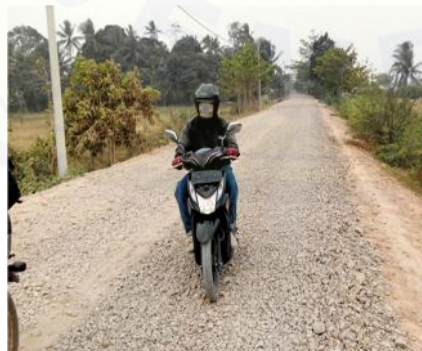
Gambar 2.19 Agregat licin
