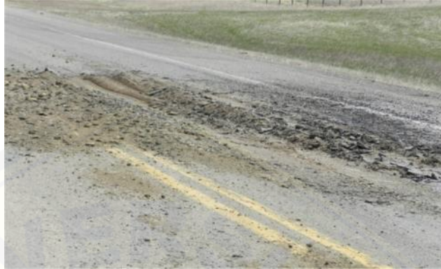
Gambar 2.16 Jembul ( upheaval )
