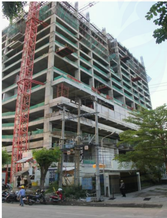
Proyek Apartement One East Residence
