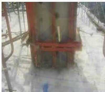
(a) Bekisting Kolom
