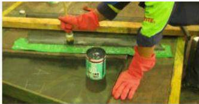
Gambar 3.11 Pelapisan Lem (Sumber: Summa Learning Center, 2001)
