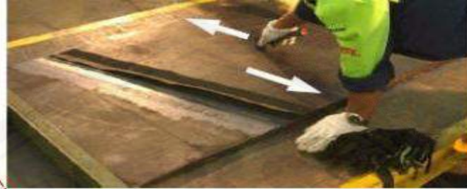
Gambar 3.12 Proses Stitching (Sumber: Summa Learning Center, 2001)
