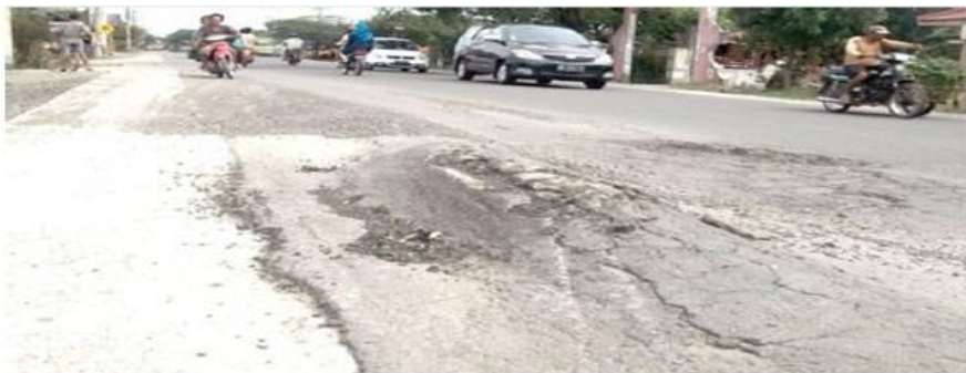
Gambar 2.20 Jembul ( upheaval )
