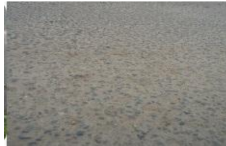
Gambar 2.24 Agregat licin
