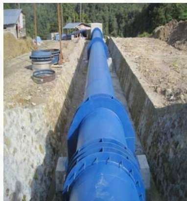
Gambar 2.5 Pipa pesat (penstock)
