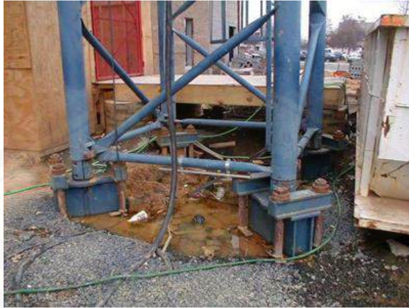
Gambar 3 Base Section Tower Crane ( from : science.howstuffworks.com )
