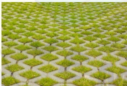
Gambar 4.42 Grass Block (Sumber: archify.com)
