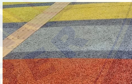
Gambar 4.43 Beton Poros (Sumber: betonporous.com)
