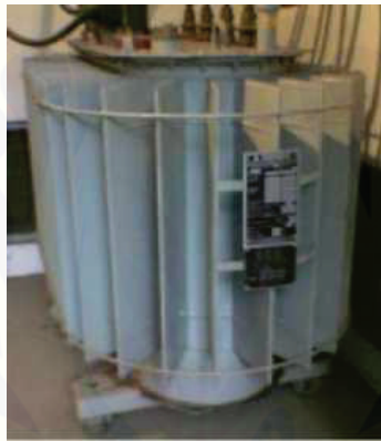
FIGURE 1. Power Transformer
