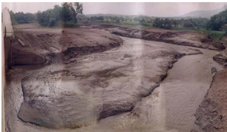
Gambar 4.1 Kondisi Flushing upstream DAM Sampean Baru
