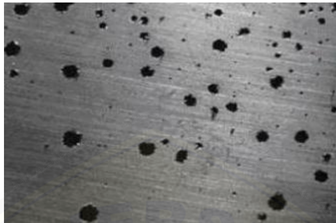
Gambar 2.6 Korosi sumuran (Utomo, 2009)
