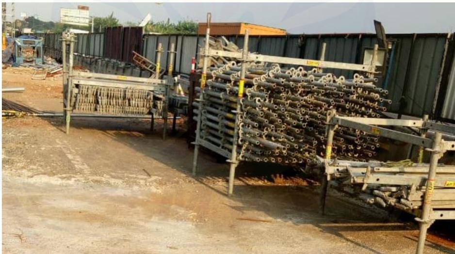
**Gambar 6.2** Peralatan shoring *pier head*.
