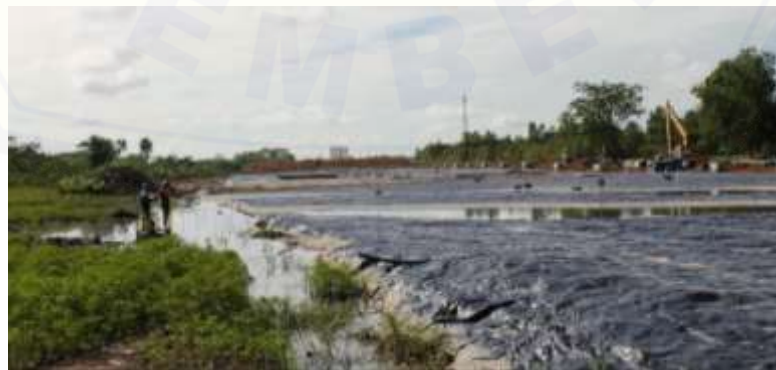
Gambar 2.6 Area Kerja Vacuum Preloading
