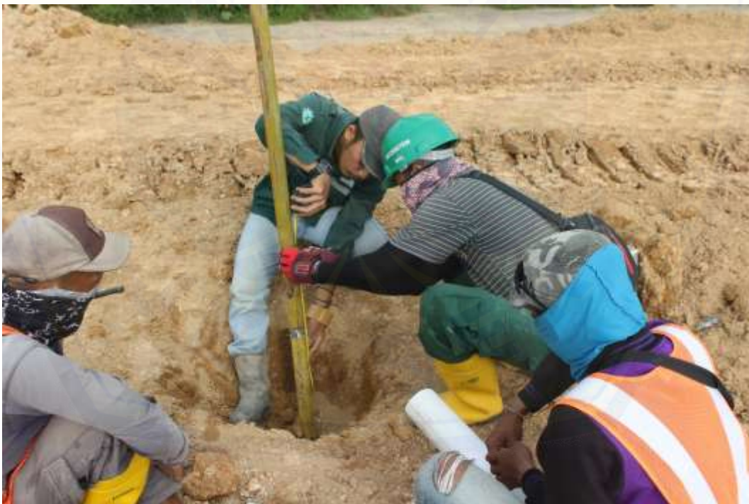
Lampiran 3 Pemasangan Settlement Plate
