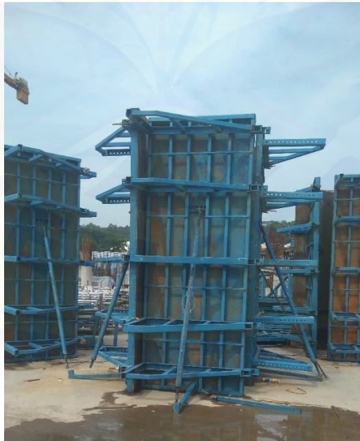
Gambar 2.1 Bekisting Sistem PT. PP presisi
