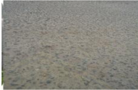
Gambar 2.19 Pengausan (Sumber: https://kerusakanjalann.blogspot.com )
