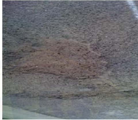
Gambar 2.17 Pelepasan Butir (Sumber: https://kerusakanjalann.blogspot.com )
