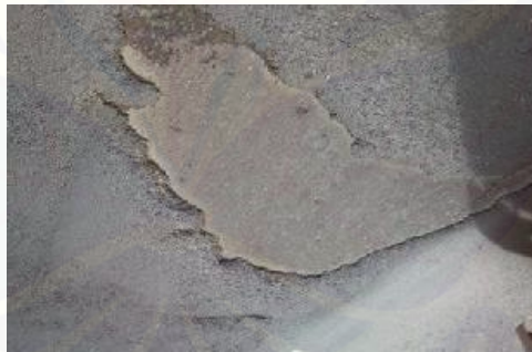
Gambar 2.18 Pengelupasan (Sumber: https://kerusakanjalann.blogspot.com )
