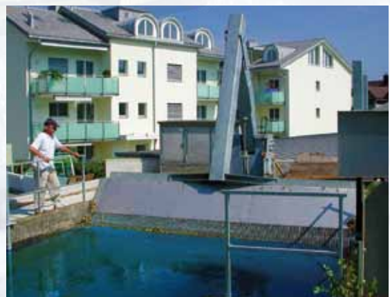
The automatic trash rack cleaner is indispensable, increasing energy production.
