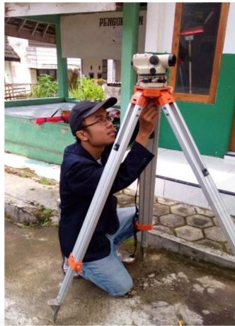
Gambar Q.7. Persiapan Alat Waterpass
