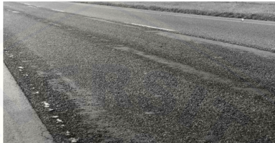
Gambar 2.21 Pengausan ( polished aggregate ) (Sumber: Google Images)
