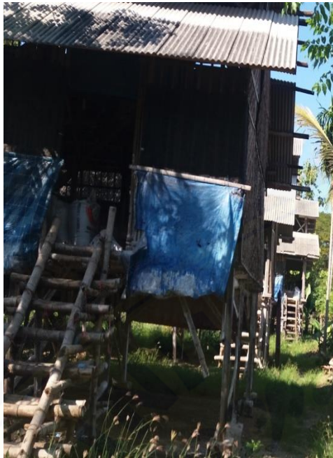
Gambar 13. Atap Kandang (Asbes)
