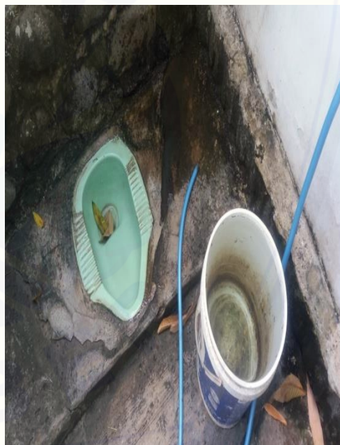
Gambar 8. Jamban Cemplung
