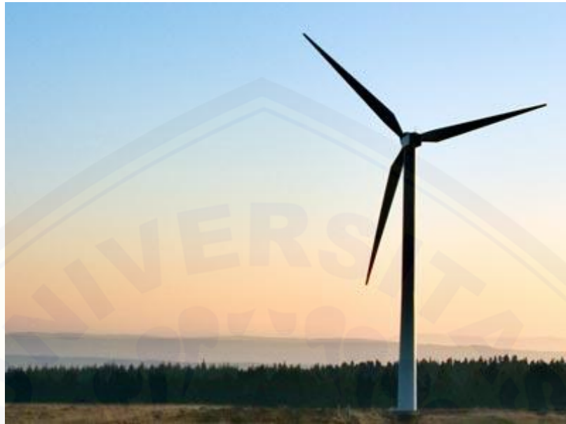
Gambar 2.5 Turbin Angin Sumbu Horizontal
