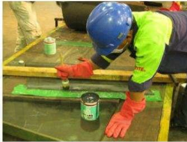
Gambar 3.13 Pelapisan lem (Sumber: Summa Learning Center )
