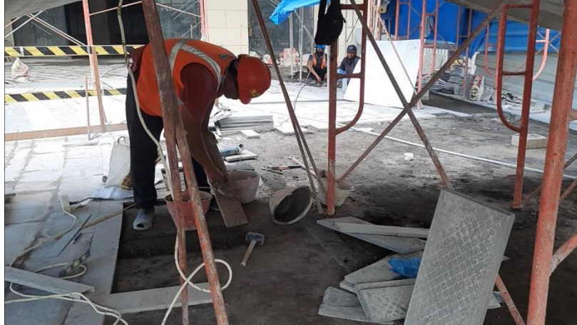
Gambar 4.4 Pemasangan Granit Connecting Bridge LT GF Ukuran (15x60) Dan (30x60)
