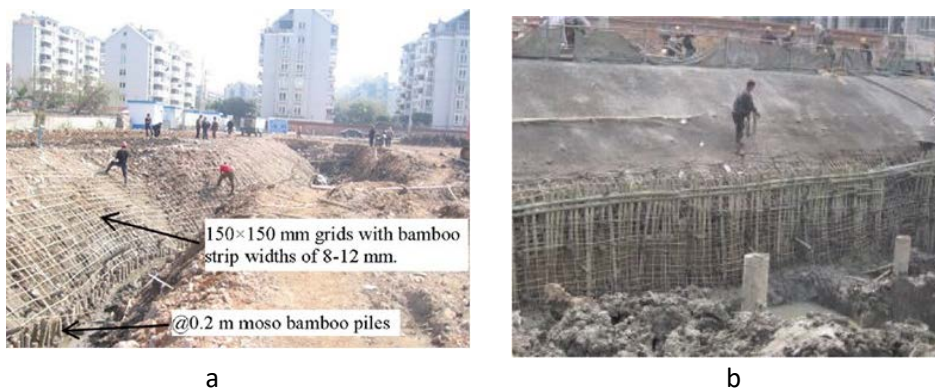
Fig. 5. Combination of bamboo soil nails, bamboo sheet piles, and bamboo reinforced shotcrete for slope stabilization (adapted from [16, 17]).
