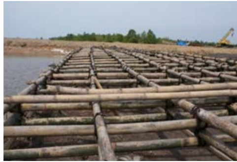
Fig. 6. Bamboo grid for soft soil reinforcement (adapted from [37]).
