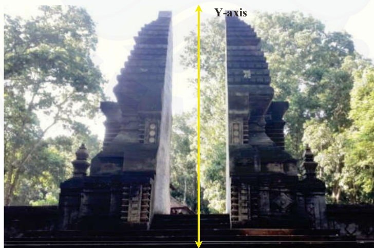
FIGURE 3. Reflection property in entrance gate
