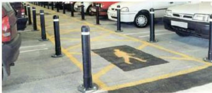
Figure 2.1 Pedestrian walkway pada area parkir kendaraan. Sumber: Health and Safety Executive (2012a)
