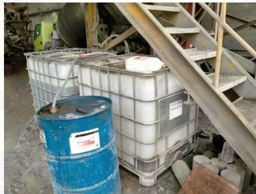
Gambar 2.5 Gambar Sistem Air Mesin Batching Plant
