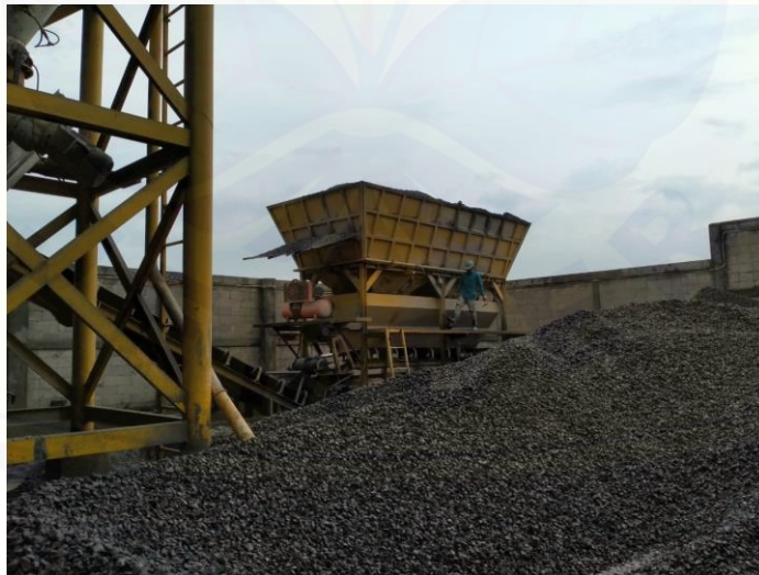
Gambar 2.3 Gambar Sistem Split dan pasir mesin Batching Plant
