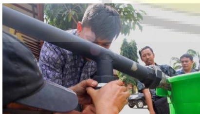
Figure 9. Condenser Installation Process
