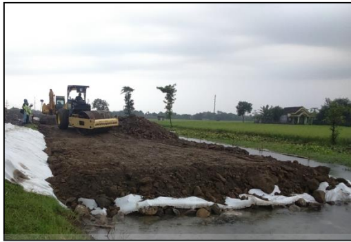
Fig 8. The Geosynthetic reinforcement applied [14]
