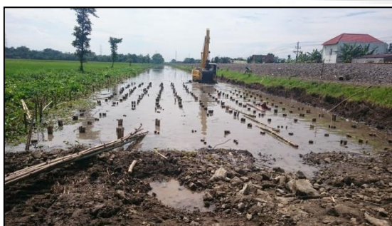
Fig 5. Driving bamboo piles [14]
