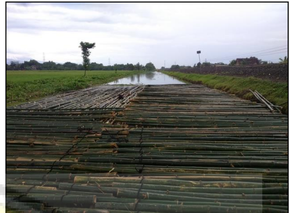
Fig 6. Installation of bamboo mattresses [14]
