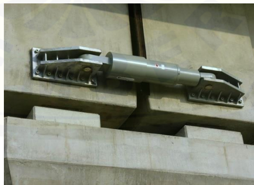
Gambar 2.15 Lock up device
