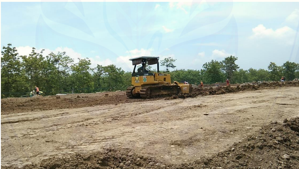
Gambar Dozer saat dozing perataan tanah
