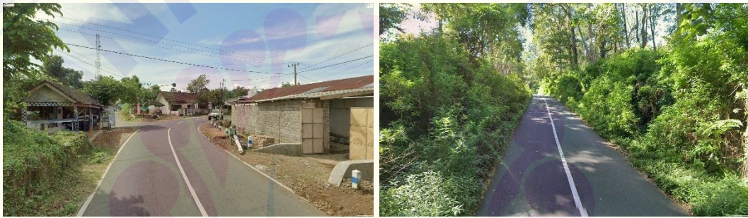
Gambar 4.5 Segmen Star Rating 3 Sepeda Motor (Kiri; KM 6+000–6+100, Kanan; 29+800–29+900)
