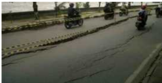
Gambar 2.14 Amblas ( grade depressions ) (Sumber : Sumantri, 2015)
