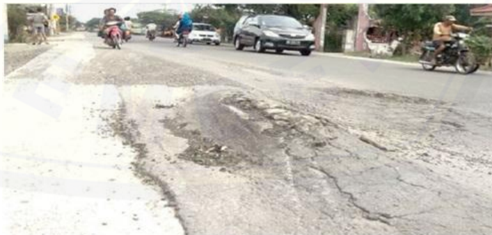
Gambar 2.20 Jembul ( upheaval )
