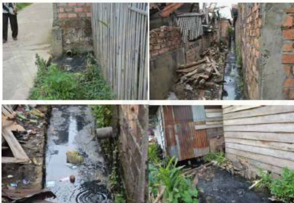
Figure 1 | Combine sewer in Palembang, Indonesia (Rachman 2020).
