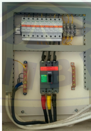
Gambar 3.4 Panel Beban AC Lantai 3
